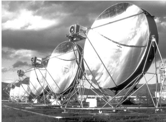
**An array of Stirling engine concentrated solar power units in Spain
